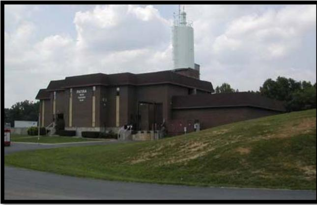
Plant 1 has a rated capacity of 3,473 gallons per minute with a net capacity of 5 million gallons per day. The main components of the treatment facility consist of the following units...
